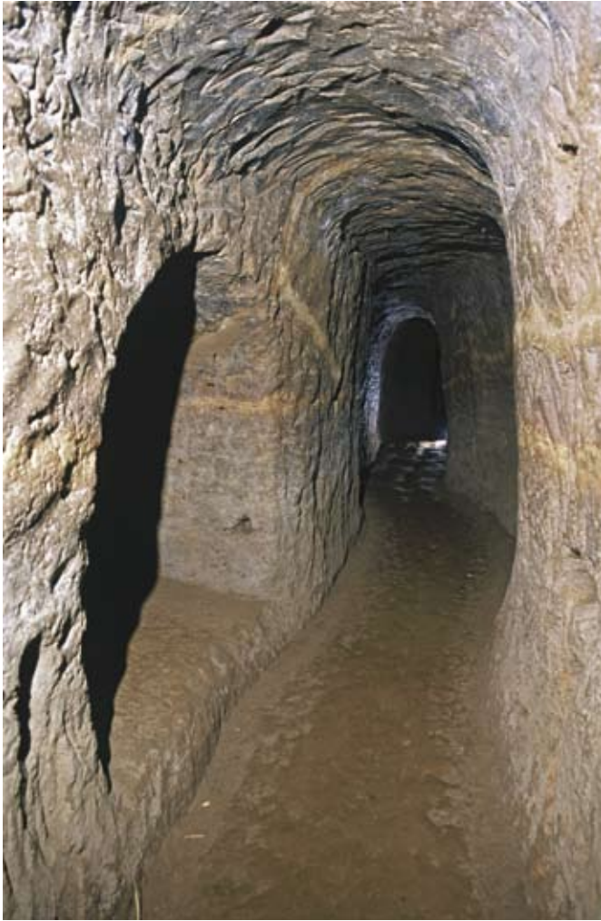
Fig. 16 - Central gallery that gives access to rooms located on each side, intermediate level of the village underground refuge of Vinh Moc, Vietnam. Height: 1,80 m (photo J. & L. Triolet).
