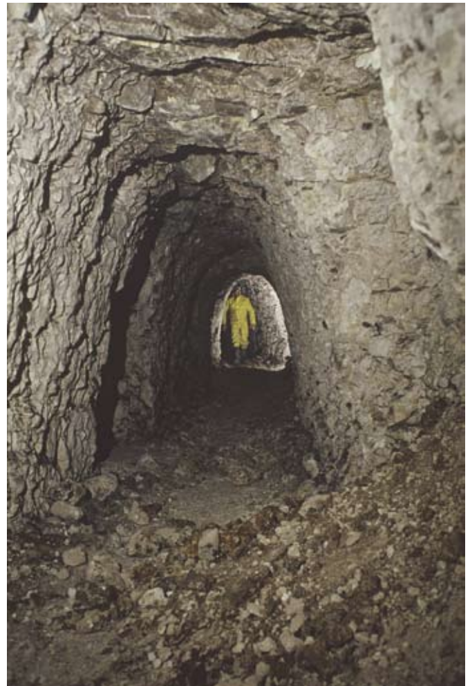
Fig. 13 - The central gallery with rooms on each side, village underground refuge of Hiermont, region of Amiens, France (photo J. & L. Triolet).
