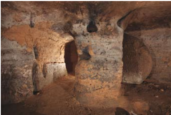
Fig. 9 - Stone door kept in its position by a rocky pillar, village underground refuge of Göstesin, Cappadocia. Diameter of the door: 1,4 m (photo J. & L. Triolet).
